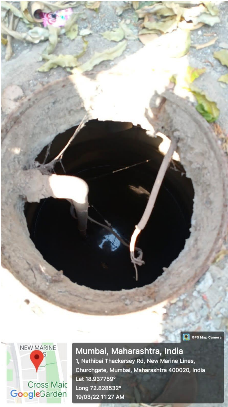
Rain water harvesting system at SNDTWU, Churchgate Campus
